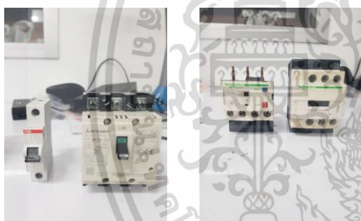
Figure 4. The example of equipment in MDB to start three phase motor consisted of breaker, No fuse breaker, relay and magnetic contactor (from the left to right)
