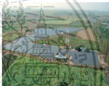
Fig. 1. 1.948 MWp a-Si thin film PV power plants installed in south part of Thailand (Prajauabkirikan province).
