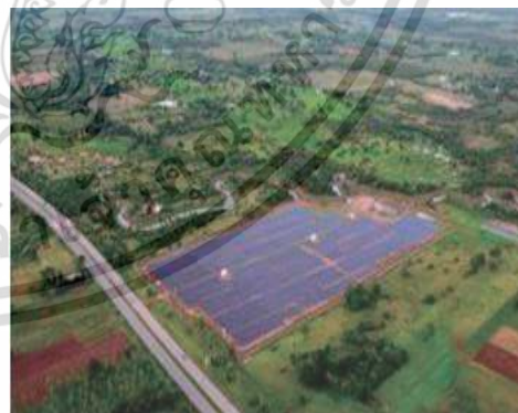
Fig. 2. 2.225 MWp a-Si thin film PV power plants installed in central part of Thailand (Lopburi province)
