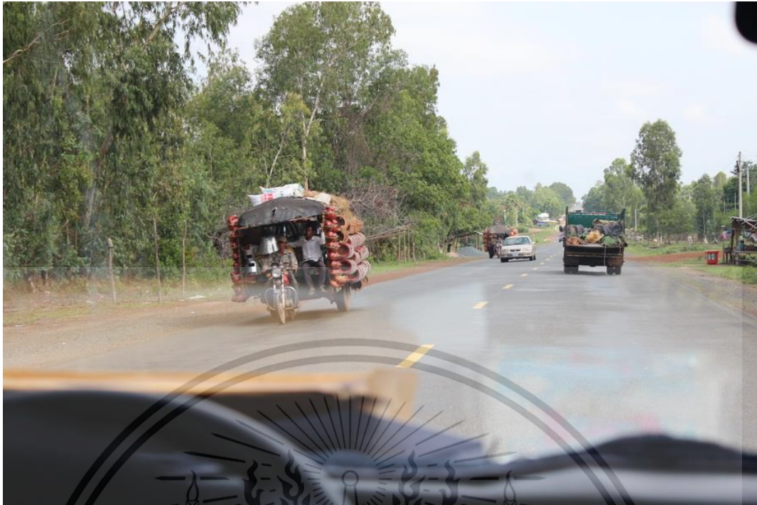
Figure 5-5. Road condition on National no.5 road in Cambodia
