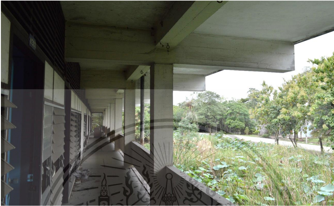
Fig. 23 Deep cantilever in Thai vocational school in Ladkrabang (Photo by the author)
