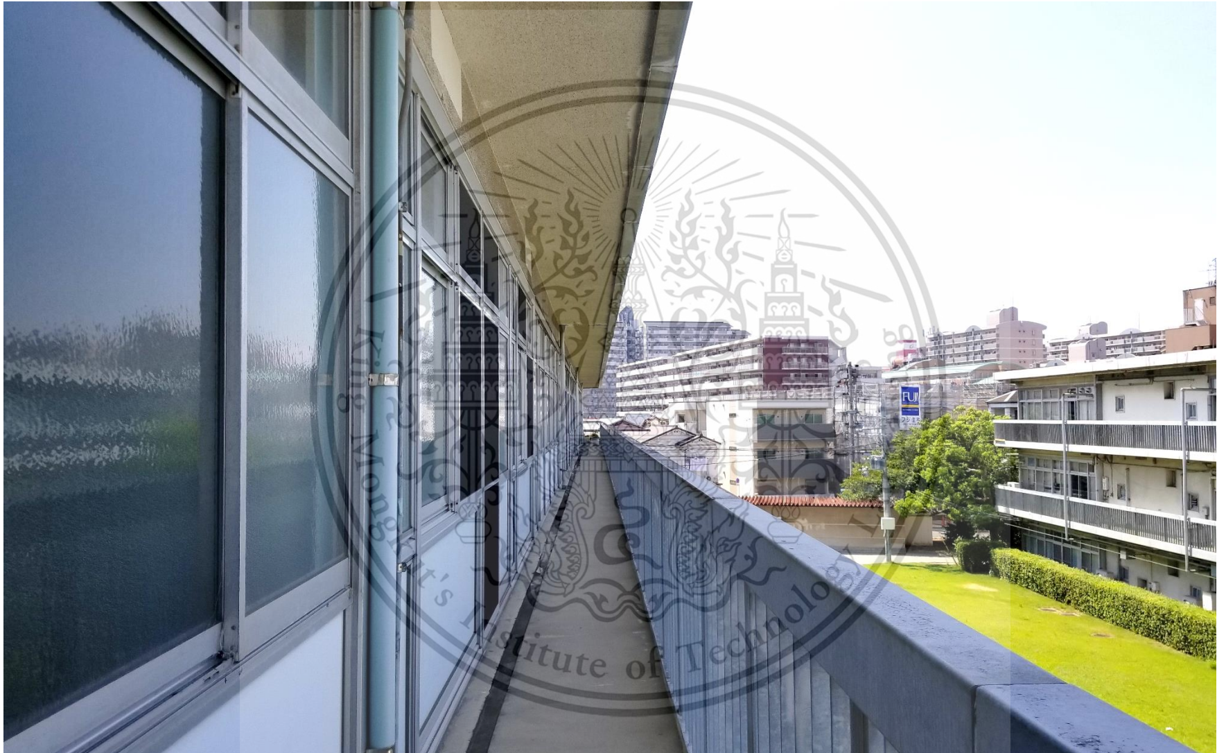
Fig. 62 South side velanda (Photo by the author)
