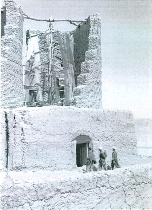
Fig. 1. Vertical axis resistance type windmill of the Sistan Basin in the border region of Iran and Afghanistan (picture taken in 1971 near Herat, Afghanistan, copyright: Alan Cookson).
