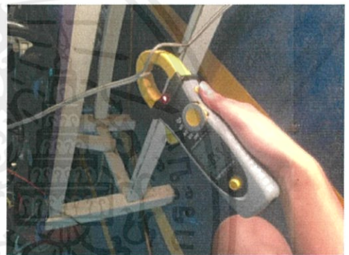
Figure 6. Measurement Electricity at 2000W and 3000W .
