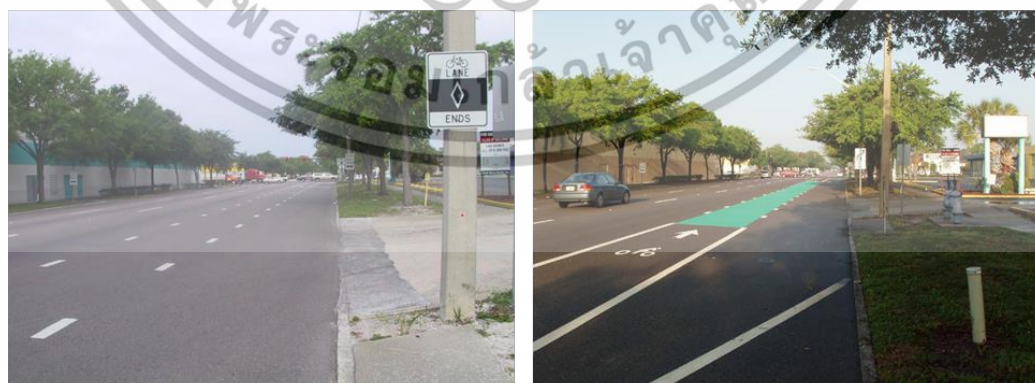
(a) Cross-section and "before" condition. (b) First "after" condition for green bike lane weaving area.
