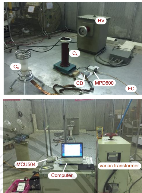
Figure 4. Test circuit set-up
