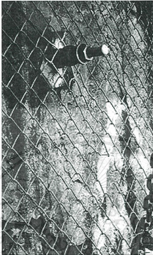
รูป 4.17 Rock bolts with wire mesh ( http://en.wikipedia.org )
