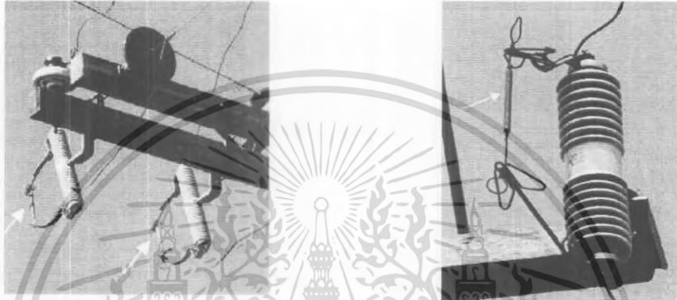
(ก) Arm Mounted Cutout with Open Link Fuse
