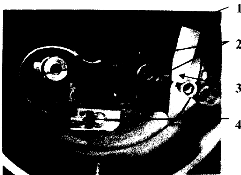
Take out heater with thermocouple
