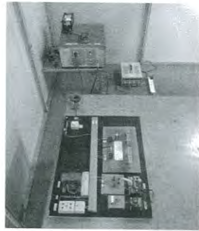
Figure 5. EMI measurement at the input of inverter
