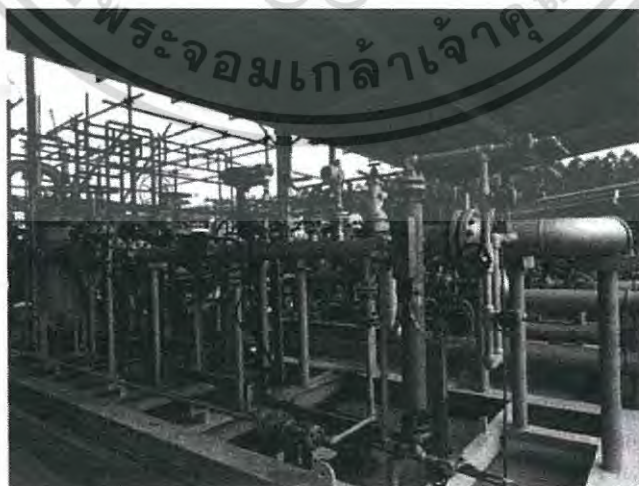
FIGURE 2. Flow metering skid for condensate residue custody transfer
