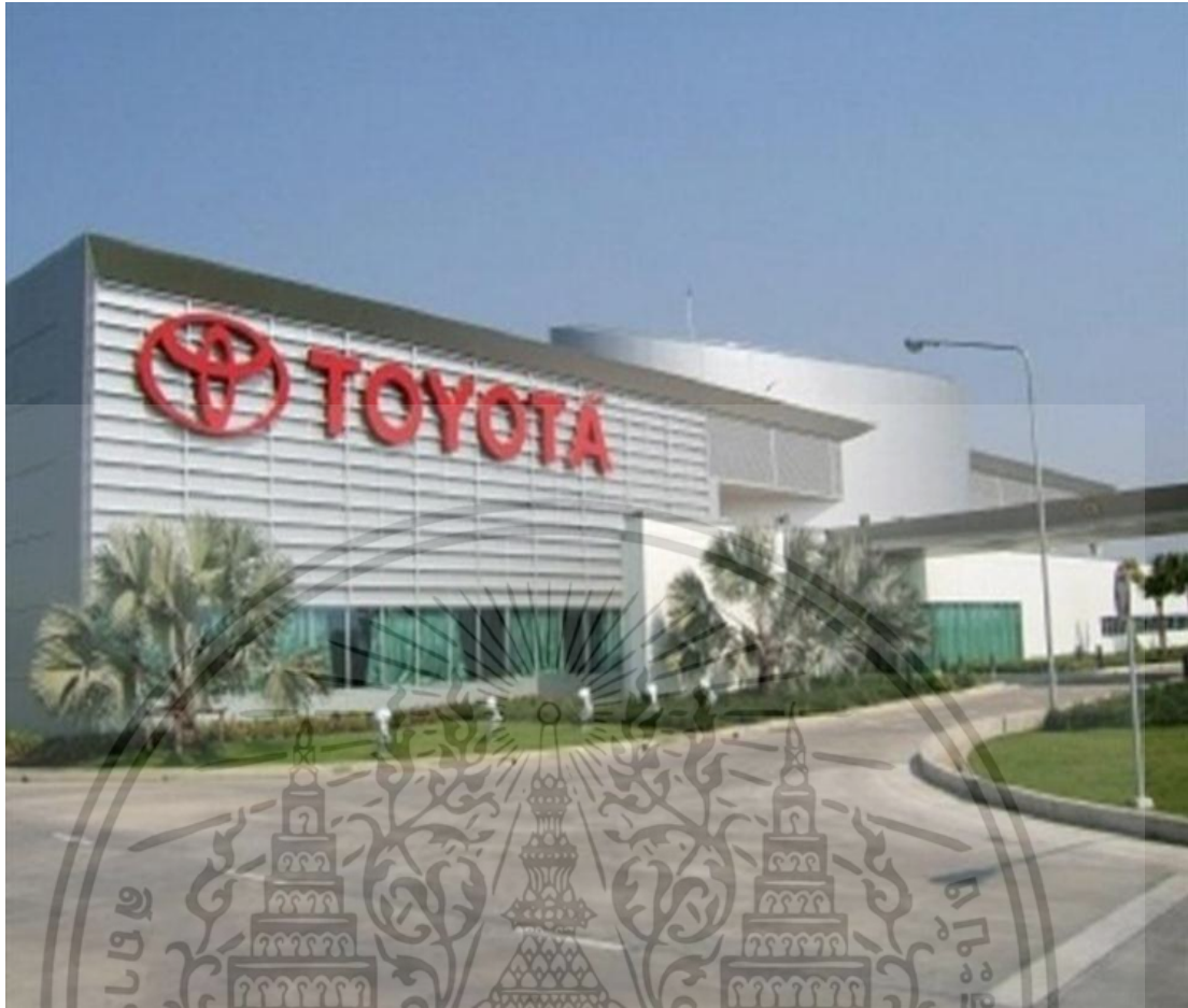
Figure 1 Toyota Motor Thailand Co. ,Ltd (Samrong Plant)
