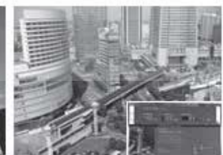
Photovoltaic power generation [moving walkway in front of Sakuragi-cho Station]
