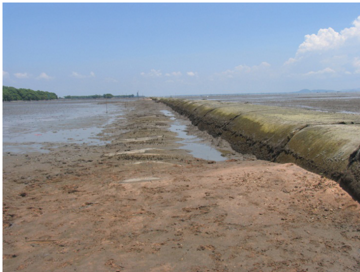
Figure 1 Sampling points and geotextile sand tube in the mud flat of the study area.
