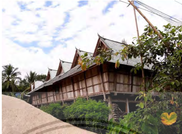
Figure 2.3 Traditional Bamboo Buildings in Xishuangbanna
