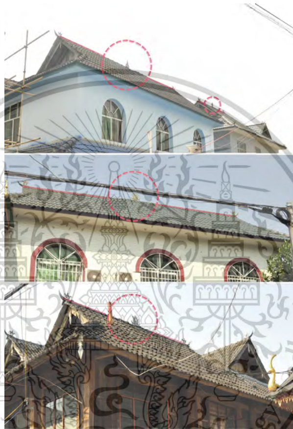
Figure 4.11 Pagoda of a temple Installed in the Middle of Principal ridge
