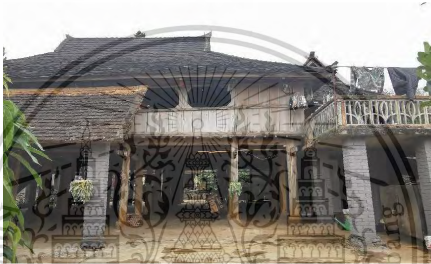
Figure 1.4 Traditional buildings in Man Yuan Village, Xishuangbanna, with building extensions (photo by author, February 2023)
