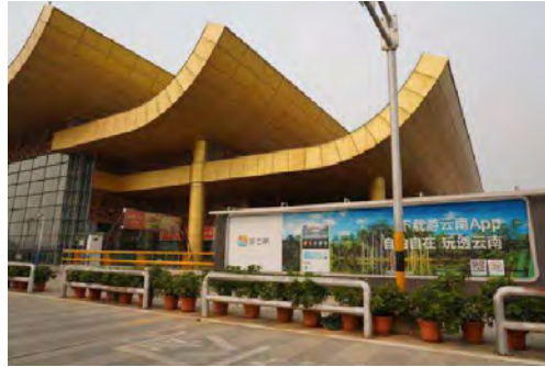
Figure 4.10 Double-eaved Roof of Xishuangbanna International Airport
