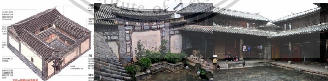
Figure 1.1 Residential buildings of the Bai nationality in Dali
