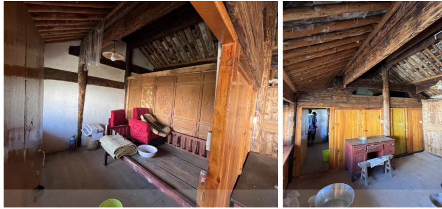
Figure 4.10 The bedroom on the first floor, positioned to the left of the shrine, is separated by wooden panels and is poorly soundproofed.
