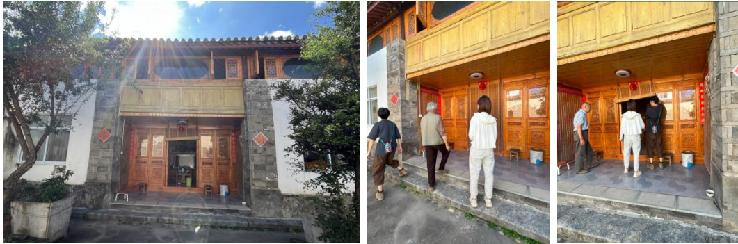
Figure 4.4 The building exterior of the old house has been renovated, the wooden structure of the house remains unchanged, mainly painting the walls, replacing windows and doors, replacing tiles
