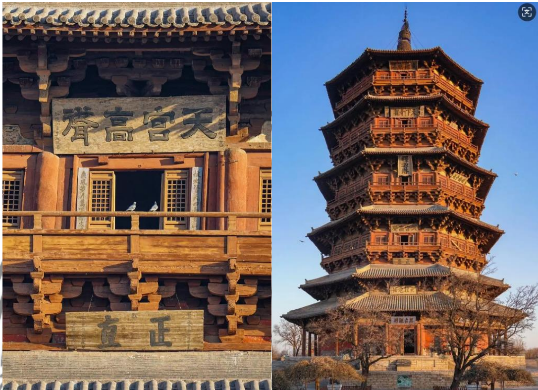
Figure 4.3 Yingxian Wood Tower Source: www.baidu.com
