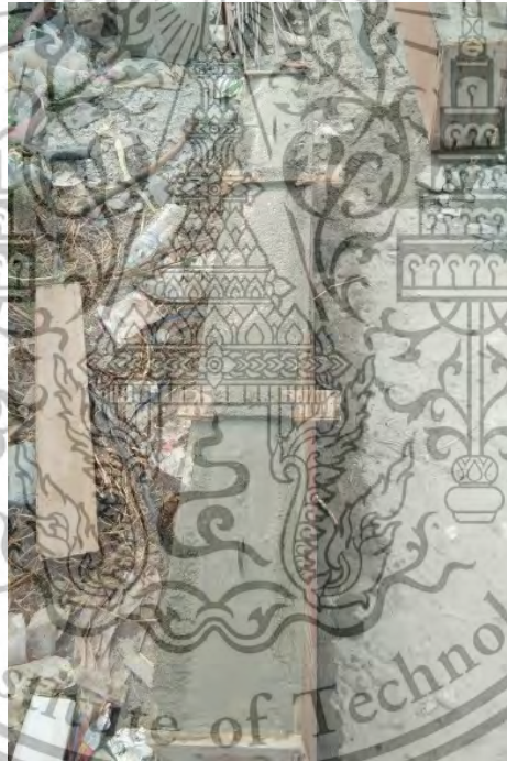
Figure 42 : Pour the concrete and have water curing after.
