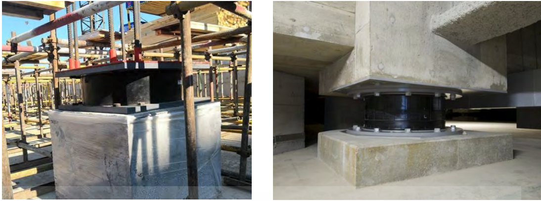
(a) During construction
