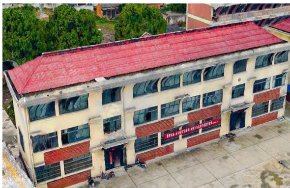
(a) Concrete structure
