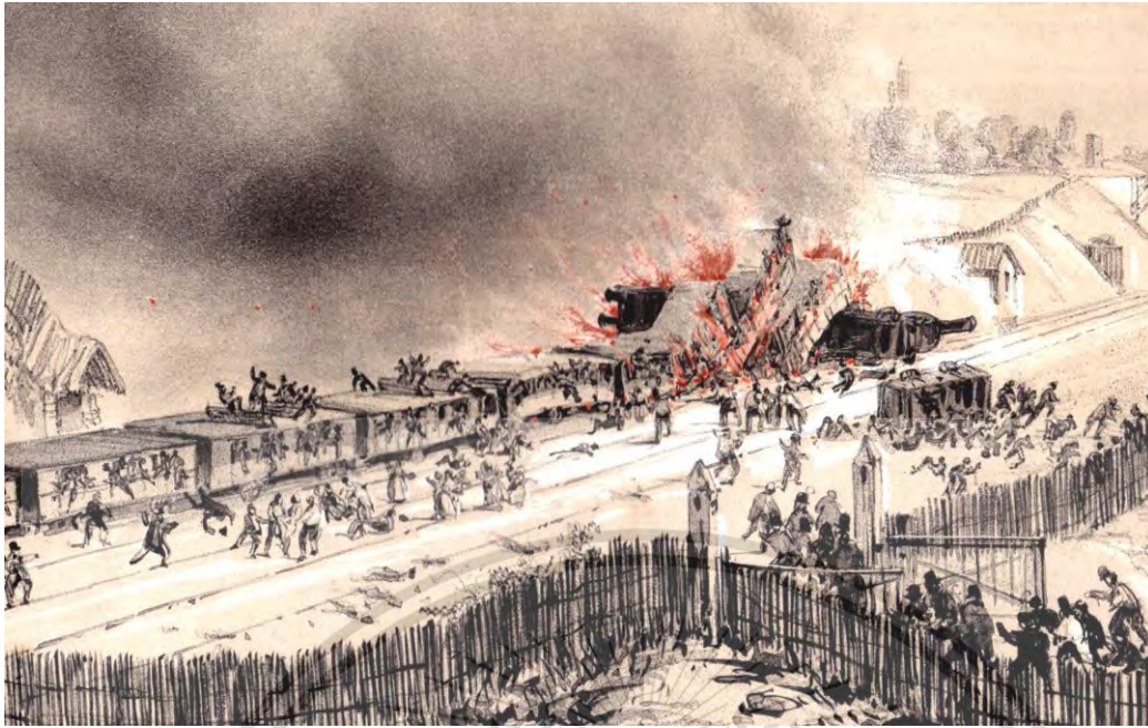
Figure 2.1 Sketch of the derailment and fire in the 1841 Versailles Train Disaster, France - the first railway accident resulting in major loss of life [3].
