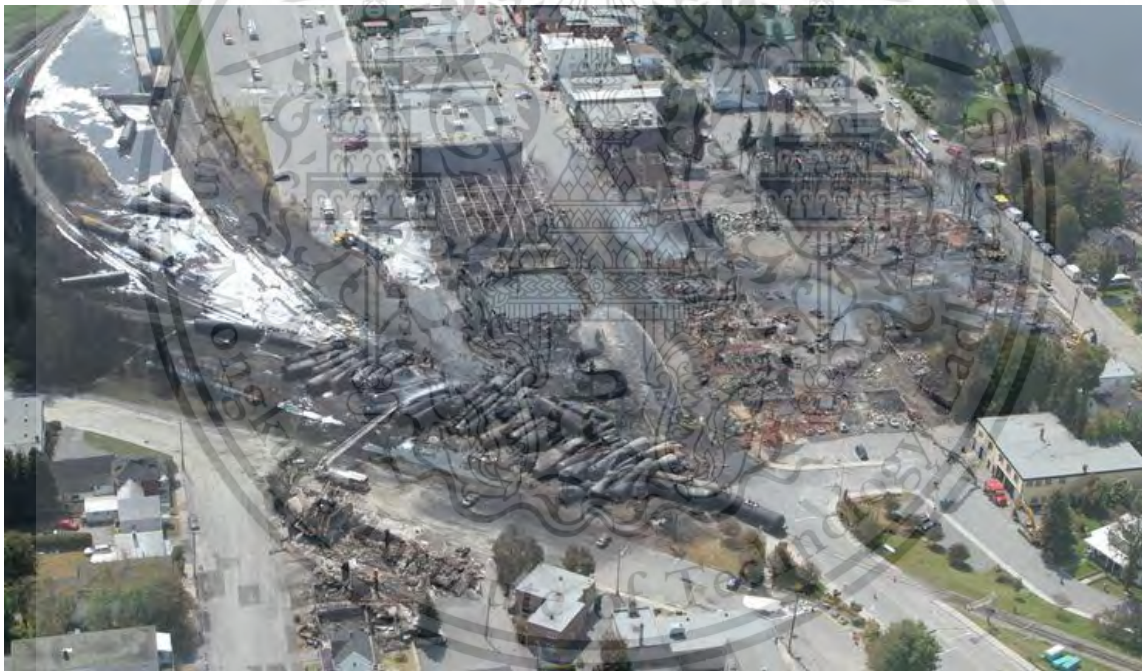
Figure 2.4 The 2013 Lac-Mégantic Train derailment and fire [6].
