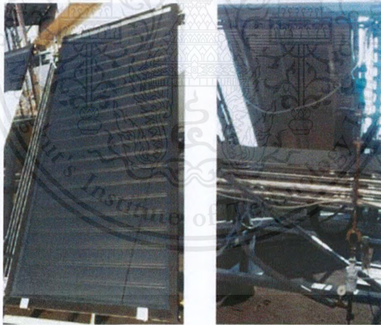
Figure 2.1 Flat plate collector [3]
