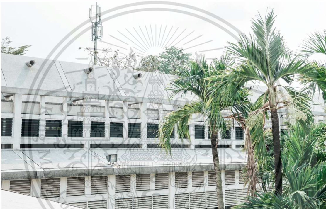
Figure 6. 1: The ventilation pipe
