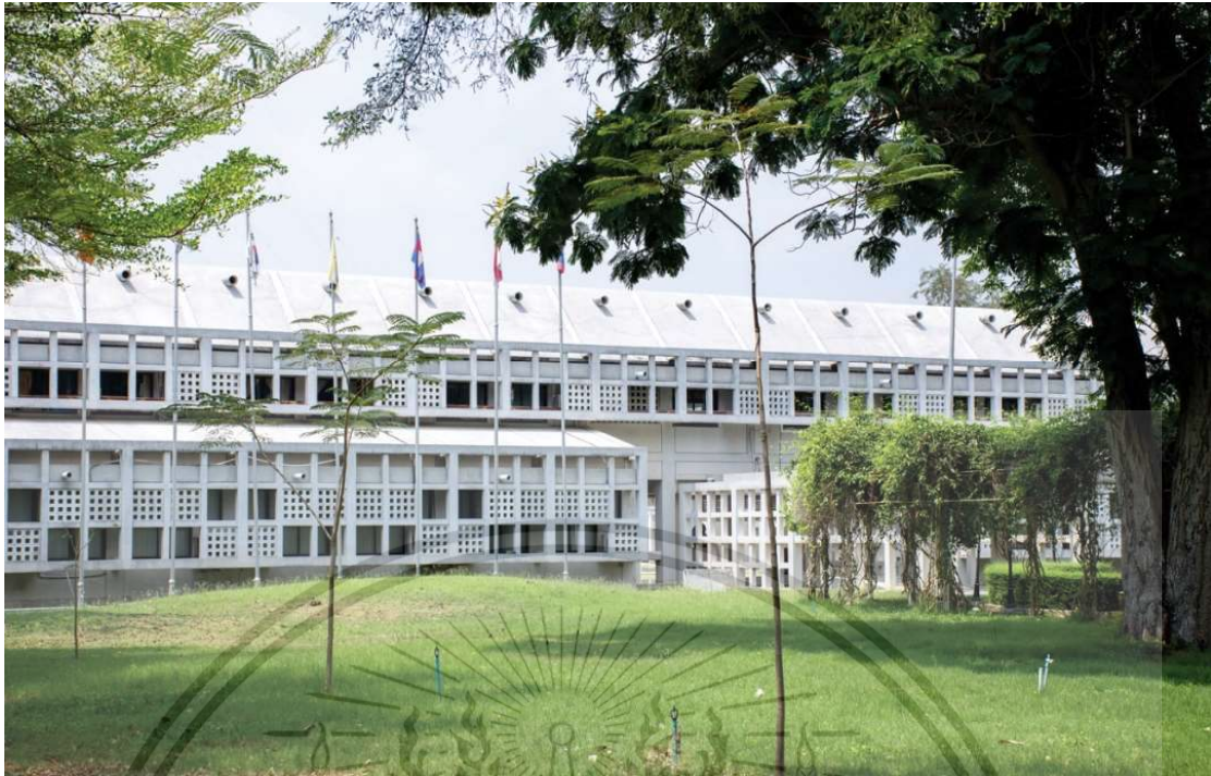
Figure 5. 4: The facade lattice
