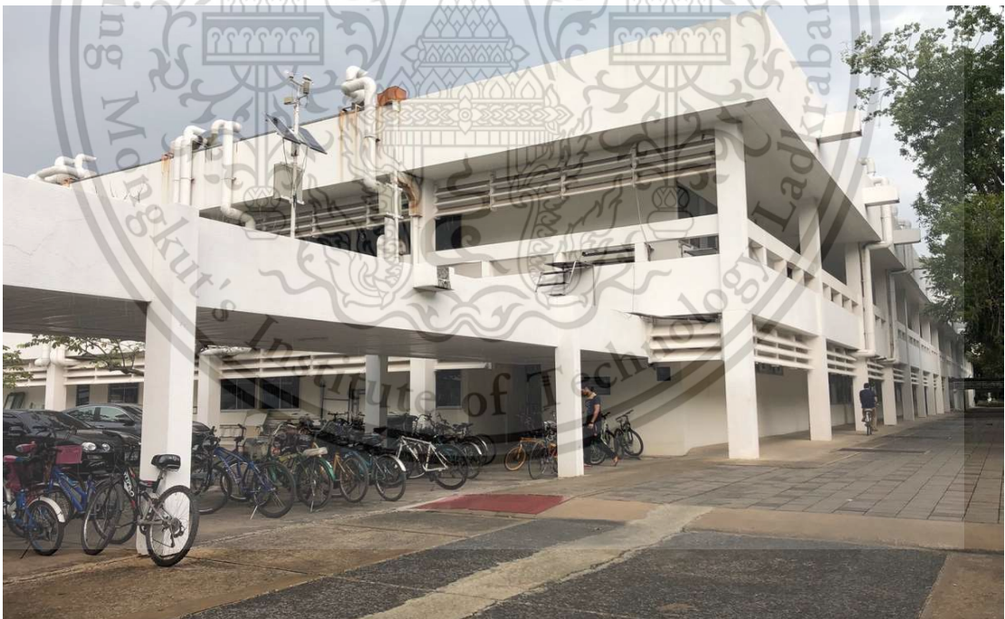
Figure 2. 7: The Asian Institute of Technology's Central Library Building (1978)
