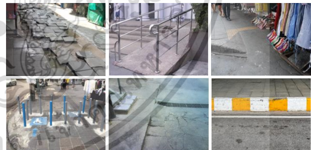
Fig. 1. Outdoor obstacles for electric wheelchair users.
