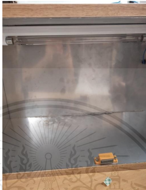
Figure 3.6 UVC light bulb installation
