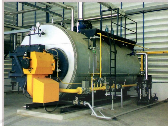
Figure 3.4 Fire tube boiler
