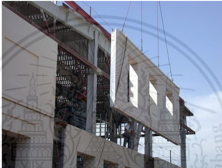
Figure 2.1 Cladding or Curtain walls
