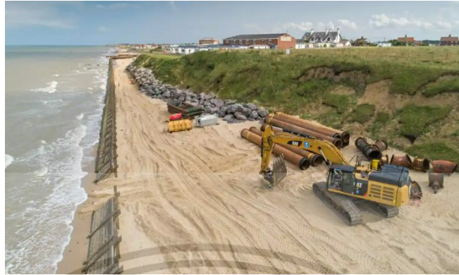
Figure 2.3 : Breach restoration [28]
