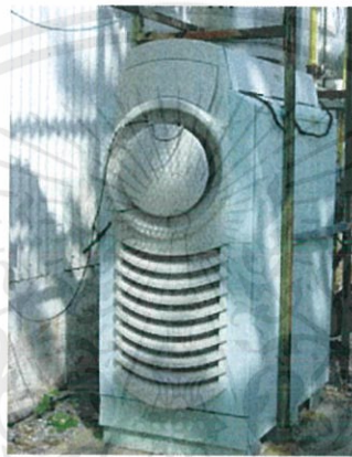
รูปที่ 2.8 A 300 kW Capstone Micro-turbine at a Demonstration Project at the Oak Ridge National Laboratory in Oak Ridge, Tennessee
