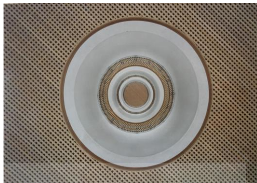
Upward view of hall on the second floor
