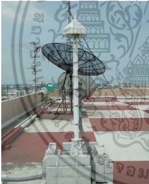
Figure 2. The dual-frequency GNSS reference station located on KMITL.
