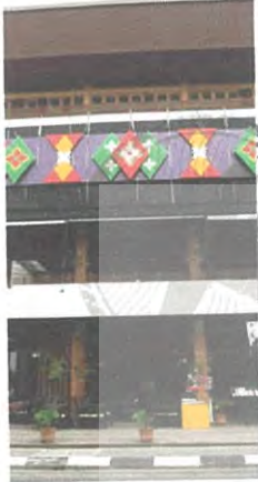
FRONT VIEW OF A BUILDING
