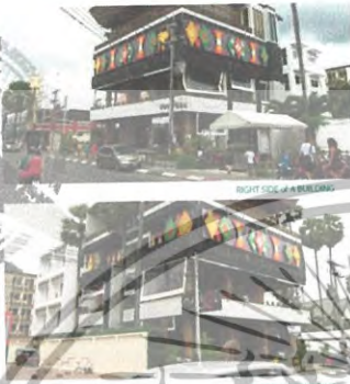
RIGHT SIDE VIEW OF A BUILDING
