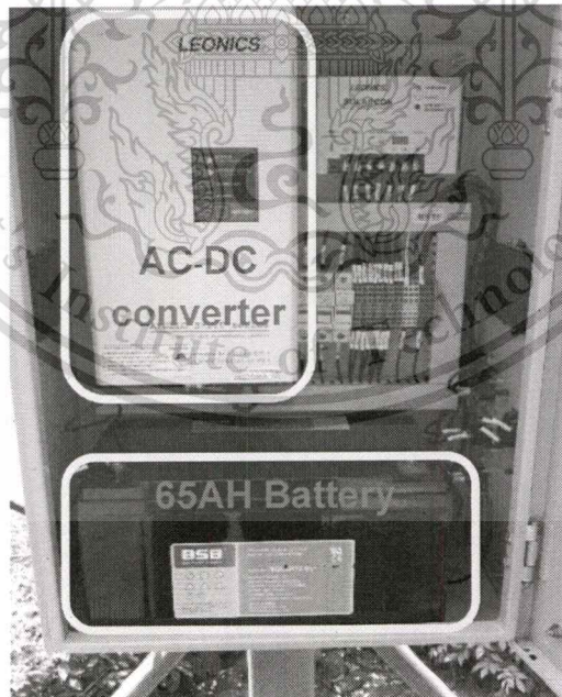
Figure 2.3: Actual hardware of the power supply unit.
