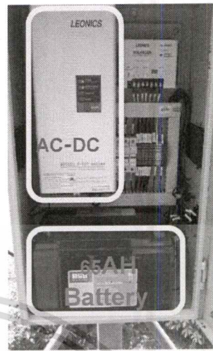
Figure 6: Actual hardware of the power supply unit.
