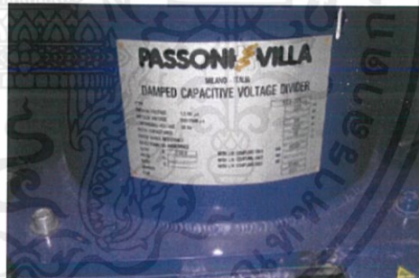
Damped Capacitive Voltage Divider (PASSONI VILLA,MILANO-ITALIA)
