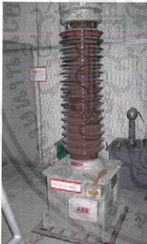
Potential Transformer (ABB Switch gear)
