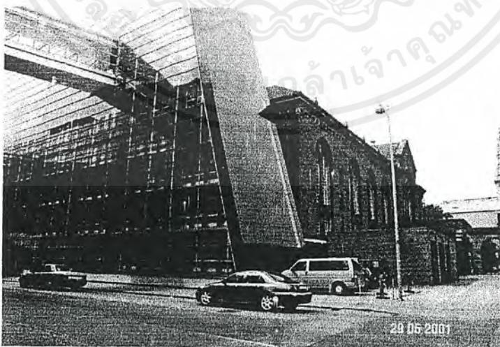
Old building connect to New Building
