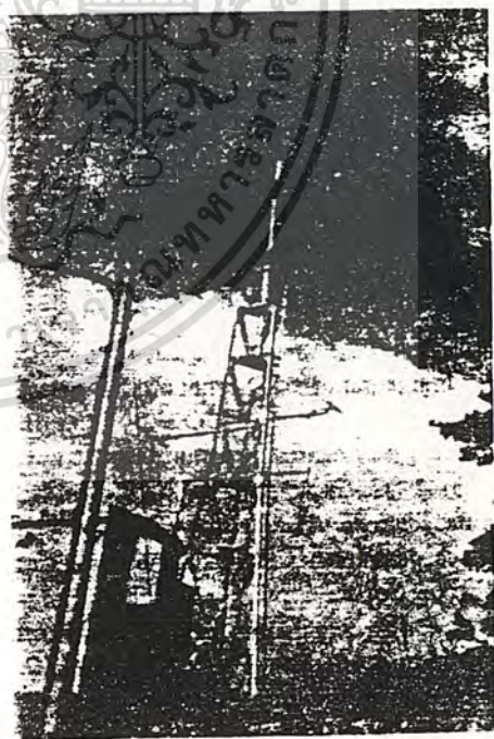
Fig. 3.29 (b) An Example of a TV Broadcast Translator Station Employing Yagi Antenna for the Transmitting Antenna
