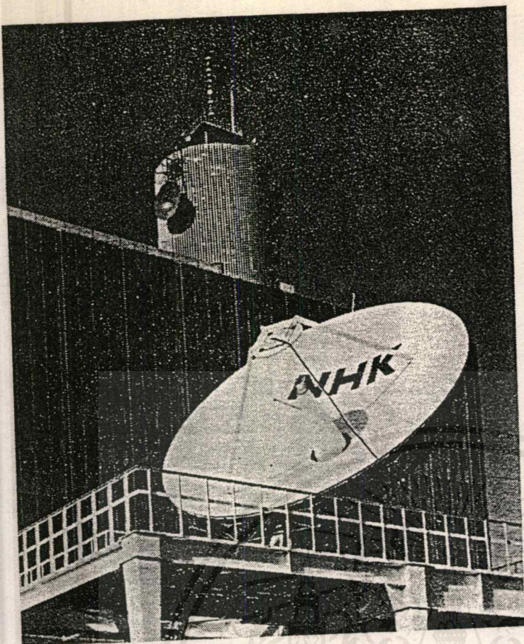
Main Earth Station
