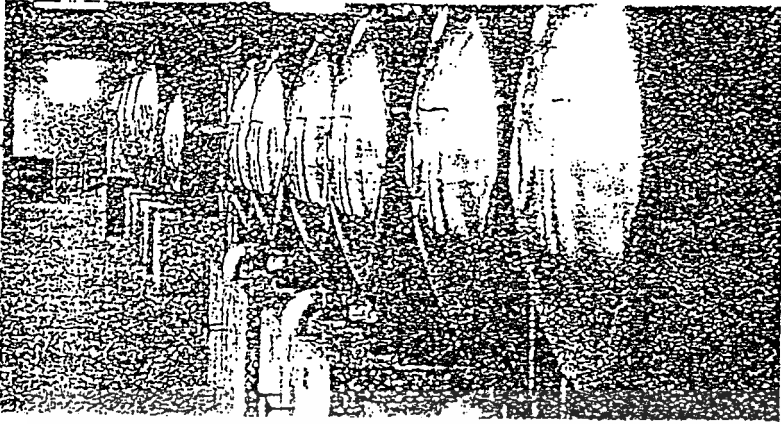
Typical tube-type generators at Choisy La Roy, France. (Courtesy of Trailgaz Ozone of America, Inc.)
